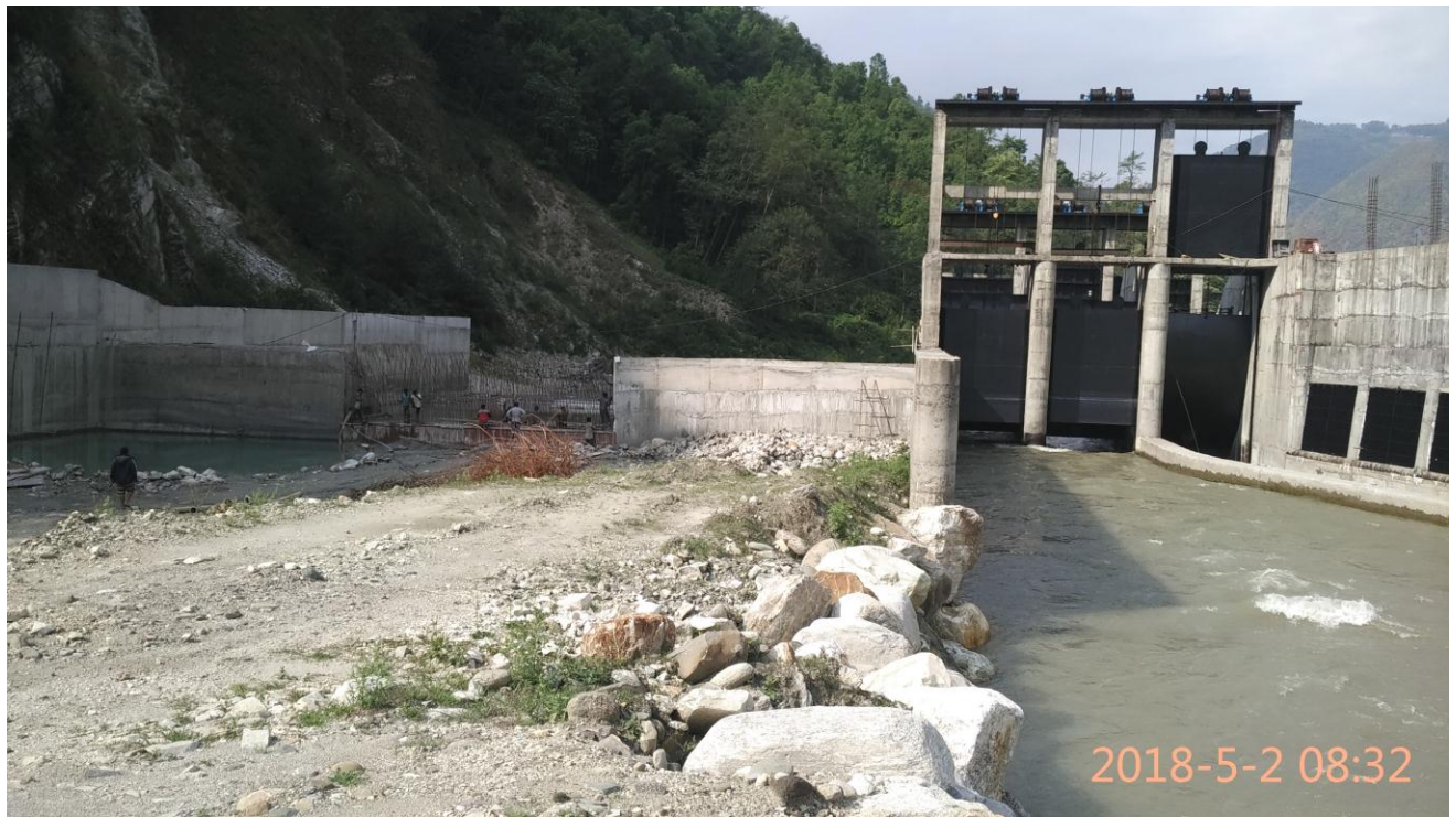
Headworks from upstream
